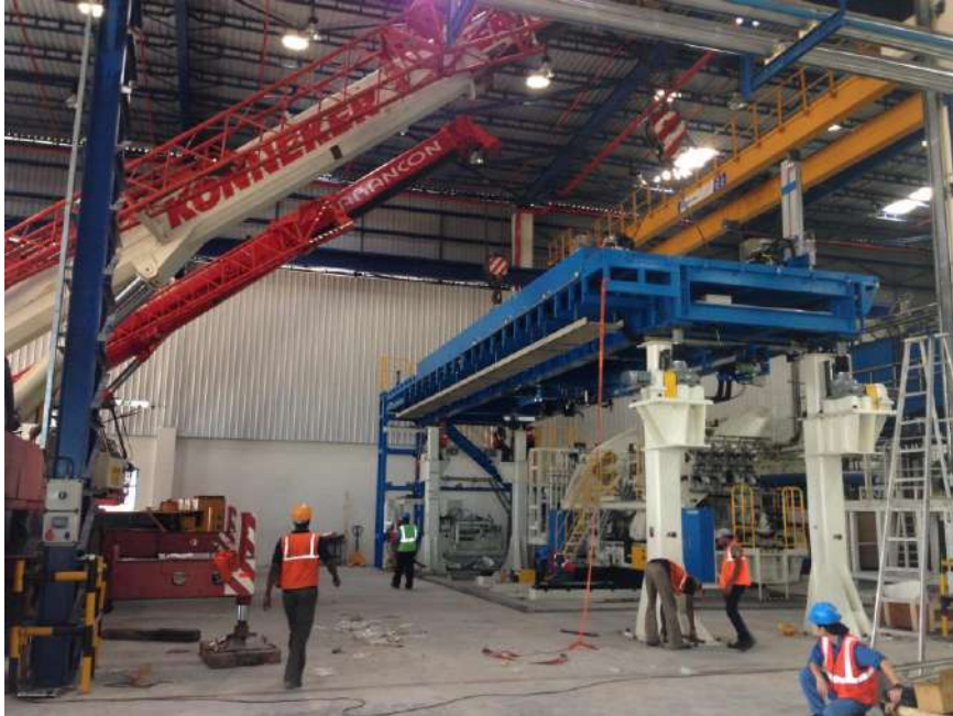
INERGY AUTOMATIVE PVT.LTD (TN) Job Type :Installation of Blow moulding machine
